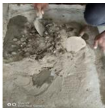
Fig 4 Mixing of concrete
