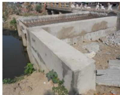
Fig.10.5 Retaining wall being constructed
