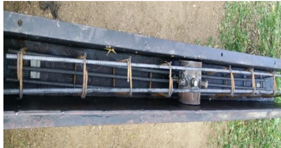
Fig 1.Reinforcement of beam with circular opening
