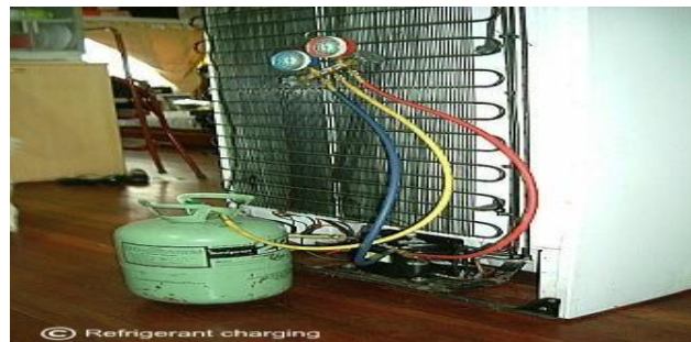
Fig Refrigerant charging
